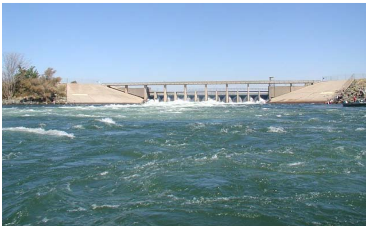
Figure 8. Photo of Thermolito Afterbay outlet on the Feather River in July 2004.
